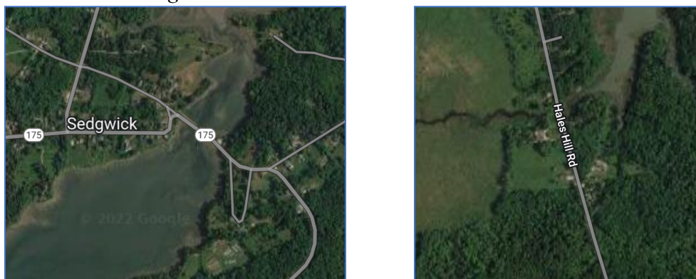
Figure M – 5: Rt. 175 Bridge and Hales Hill Road Culvert
