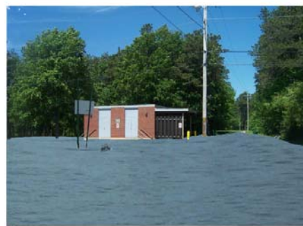
Ocean Park Route 9 sewer pump station – potential inundation, HAT + 2 ft sea level [P. Slovinsky, MGS]
